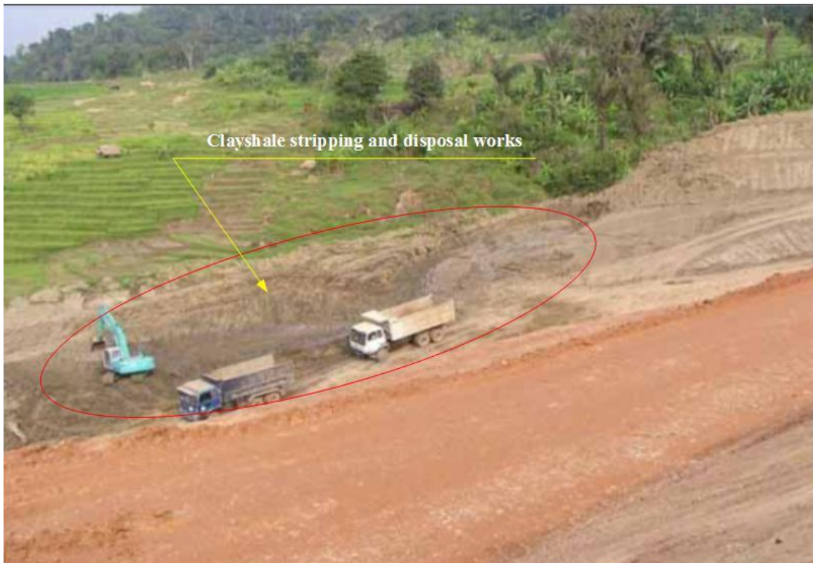
Figure 25. Stripping and disposal works for the upper layer (Jasa Marga (Persero), Tbk, 2003).
