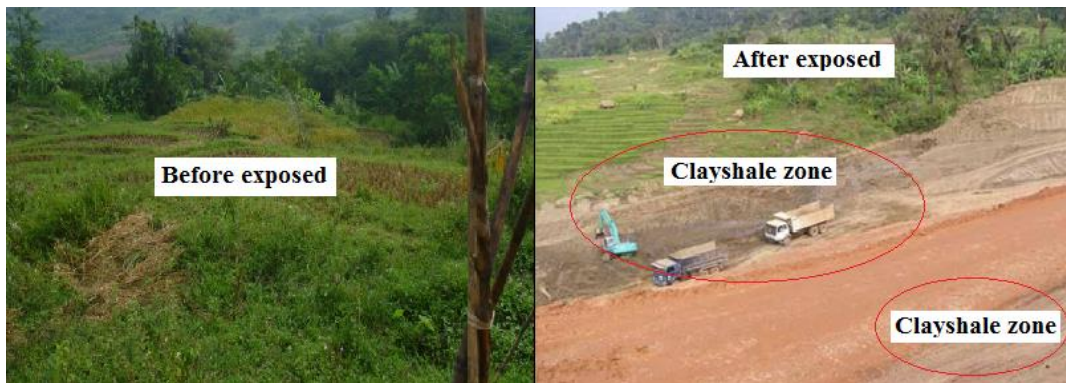
Figure 4. Clayshale in Toll Cipularang Highway (Jasa Marga (Persero), Tbk. 2003).
